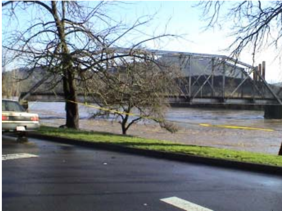
Healdsburg Railroad Bridge February 16, 2004 Peak Flow Sampling Event
