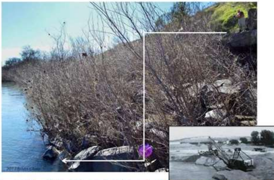
Figure 4.2.3. Channel incision at Storey Creek, a tributary in the middle of the study reach. Approximately 20-24 feet of channel incision is evident from the height difference of the concrete stabilized channel bed at the mouth of Storey Creek (upper right) that would have connected with the river bed when constructed. If not for the concrete culvert, this tributary would have incised along with the river, as did Dry Creek and other tributaries to the Russian River channel.
