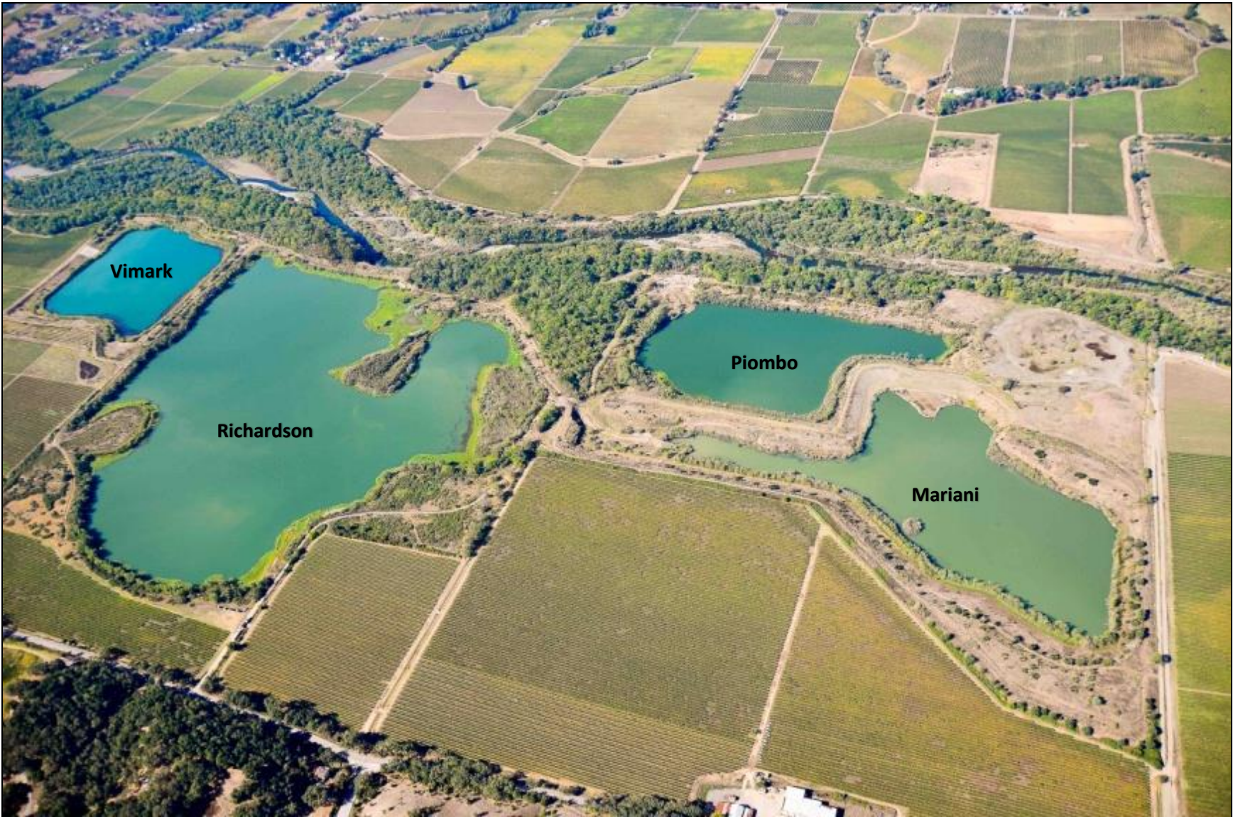
Figure C. The current configuration of the Hanson Russian River Ponds. The Hanson property consists of four ponds totaling 358 acres. Photo by Brian Cluer, NOAA Fisheries.
