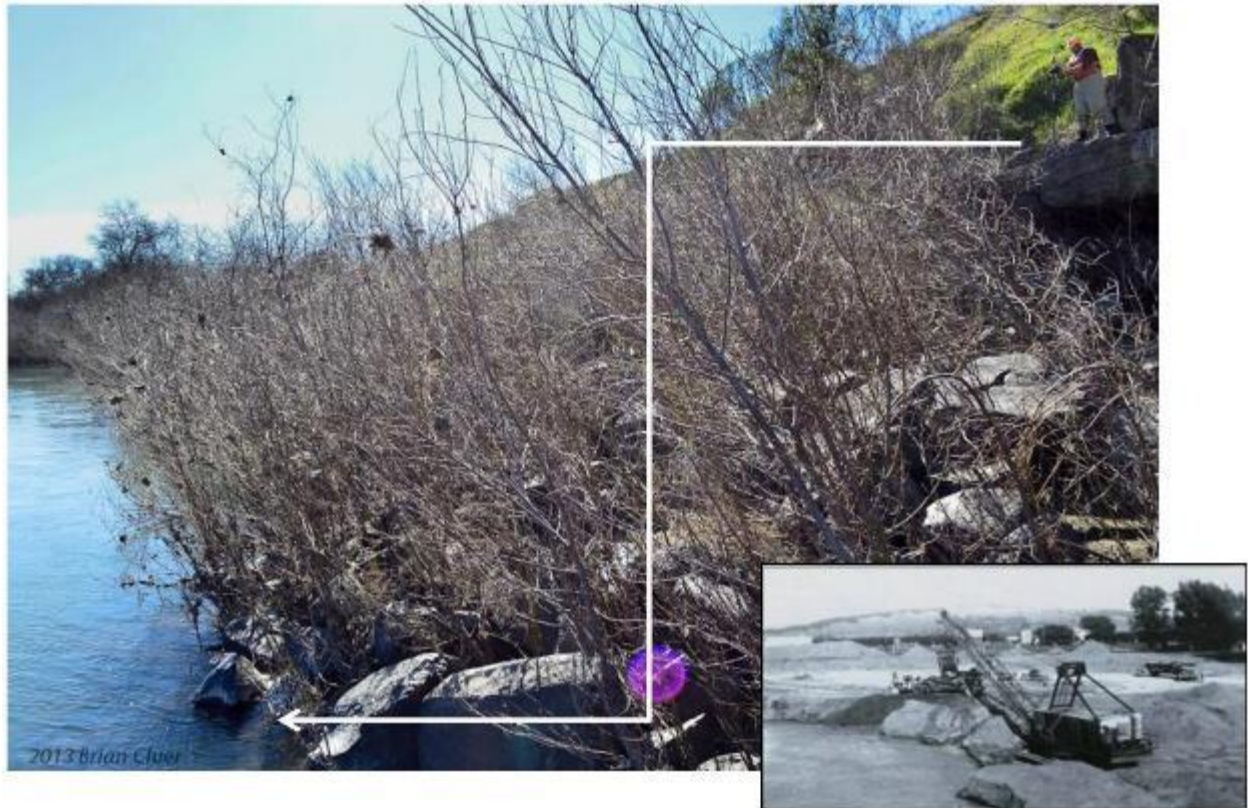
Figure 4.2.3. Channel incision at Storey Creek, a tributary in the middle of the study reach. Approximately 20-24 feet of channel incision is evident from the height difference of the concrete stabilized channel bed at the mouth of Storey Creek (upper right) that would have connected with the river bed when constructed. If not for the concrete culvert, this tributary would have incised along with the river, as did Dry Creek and other tributaries to the Russian River channel.
