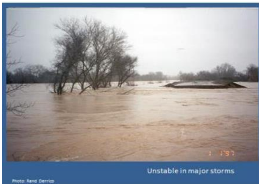
Figure 4.2.4. Levee washout at Syar ponds. Washout of the levee dividing the river (left) and one of the Syar gravel ponds in 1997.
